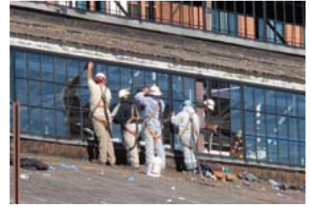
Workers installing new windows at the Boilermaker Shops
