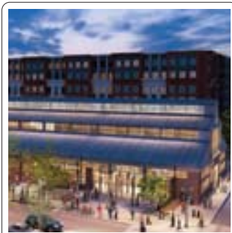
30. BOILERMAKER SHOPS 45,500 SF
