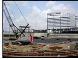
Nations Park Under Construction
