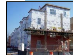
Capitol Quarter Townhomes Under Construction
